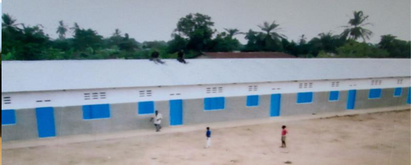
Completed "on budget - on time" May 2015
