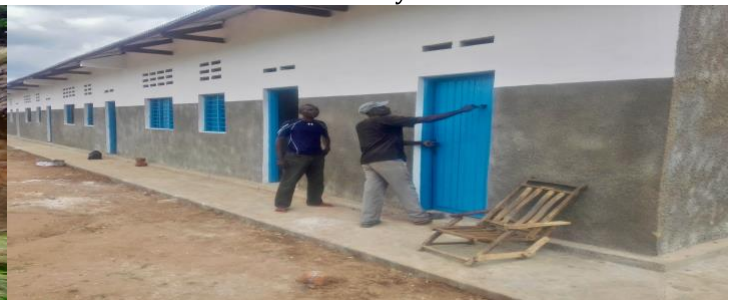
Completed "on budget - on time" January 2020
