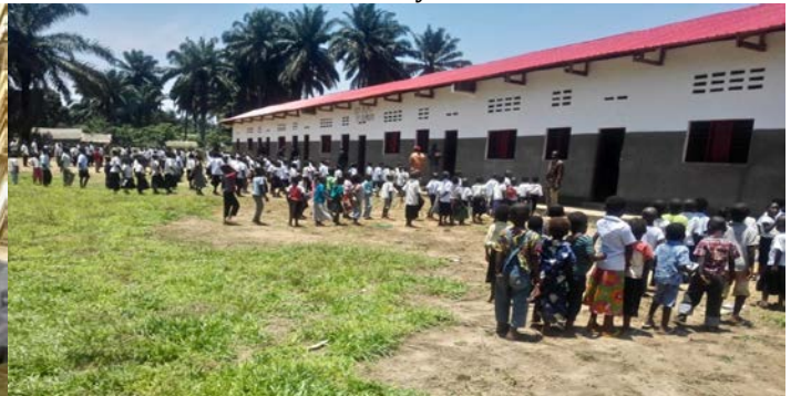
Completed "on budget - on time" September 2018
